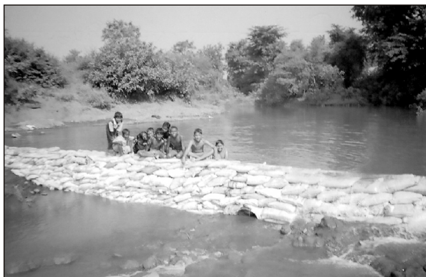
Fig. 4. Vanrai bandhara constructed by agriculture officer in Pusad block
