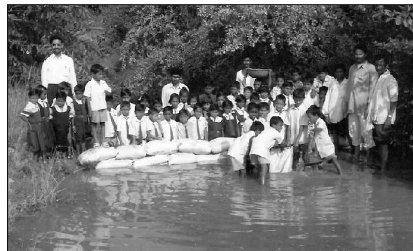
Fig. 3. Vanrai bandhara constructed by school children in Umarkhed block
