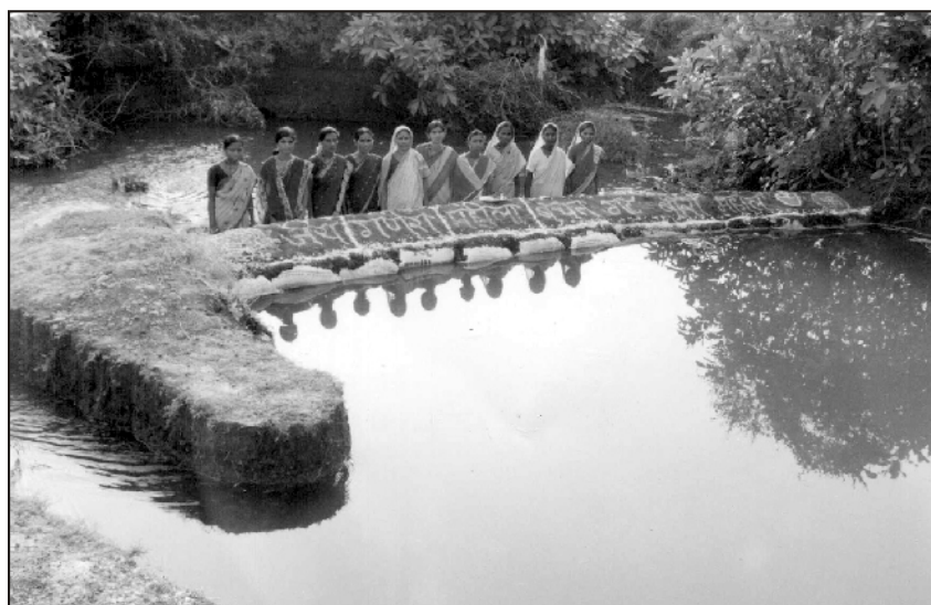
Fig. 7. Vanrai bandhara constructed by a Women SHG in Kalamb block.
