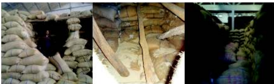
Picture 3. Hollow Formations in Stacks at (L to R) FSDs of Dhamora, Roza and Harduagunj, in UP
