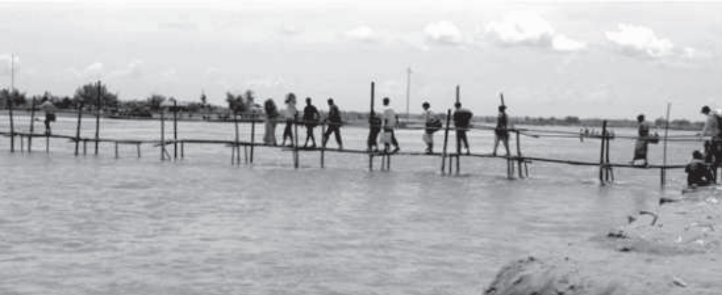
Figure 4: Temporary Bamboo Bridge over Gainadi
