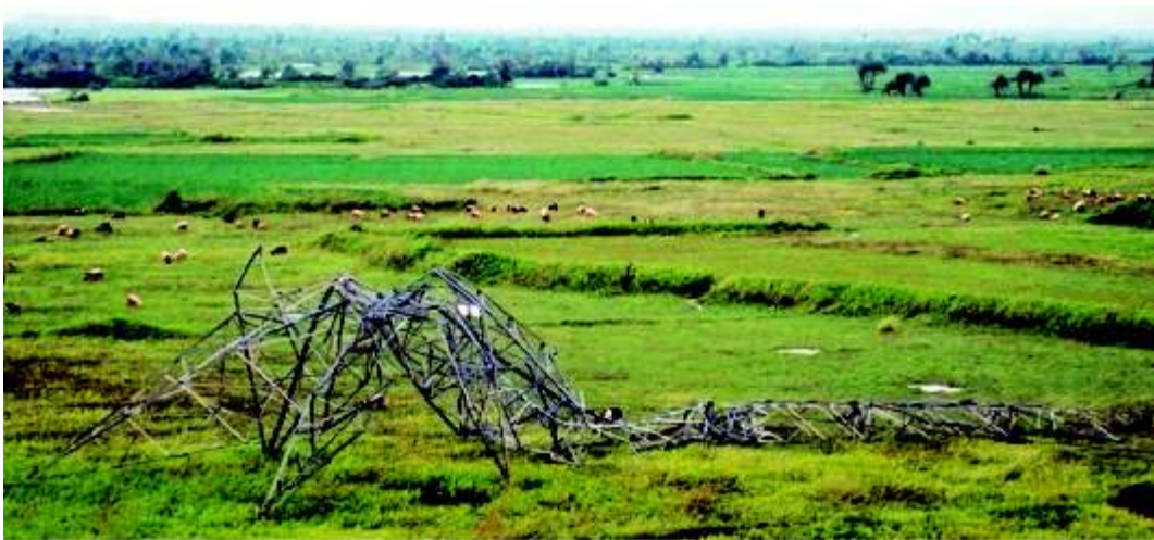
Electricity infrastructure in the district was heavily damaged by the cyclone
