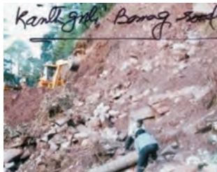
Road repairs after landslide
