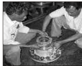
Fig 16- Application of Gasket Sealant
